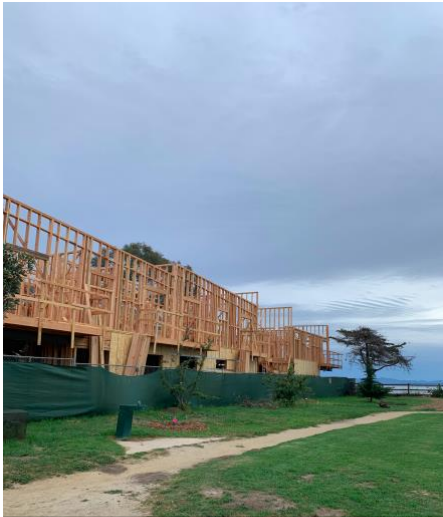
Cliff erosion has not dissuaded new development projects
